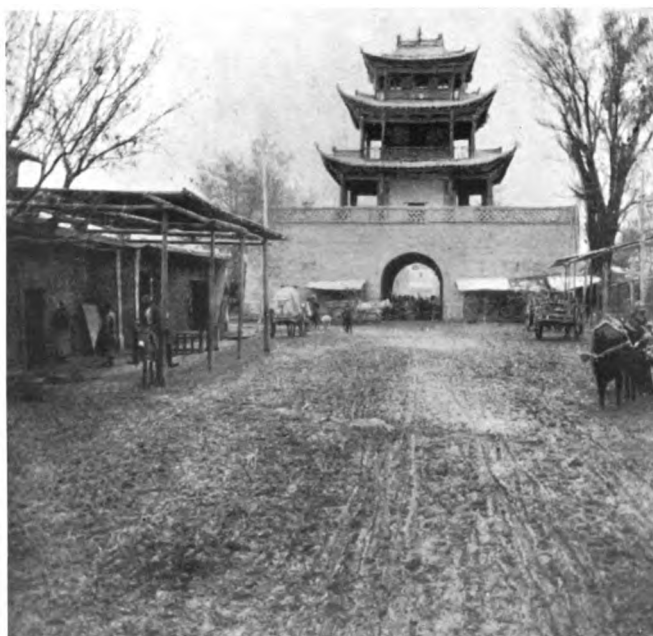
GATE IN NEW SWITING
